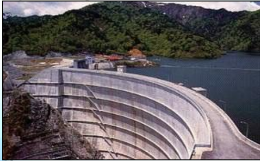
Yagisawa Dam (Arch Concrete Dam)
